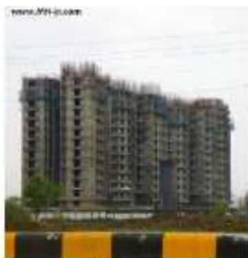
Figure 2.2: Buildings under construction MIHAN
