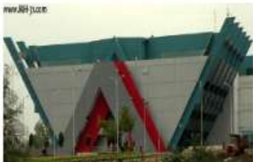
Figure 2.3: MIHAN Administrative Office
