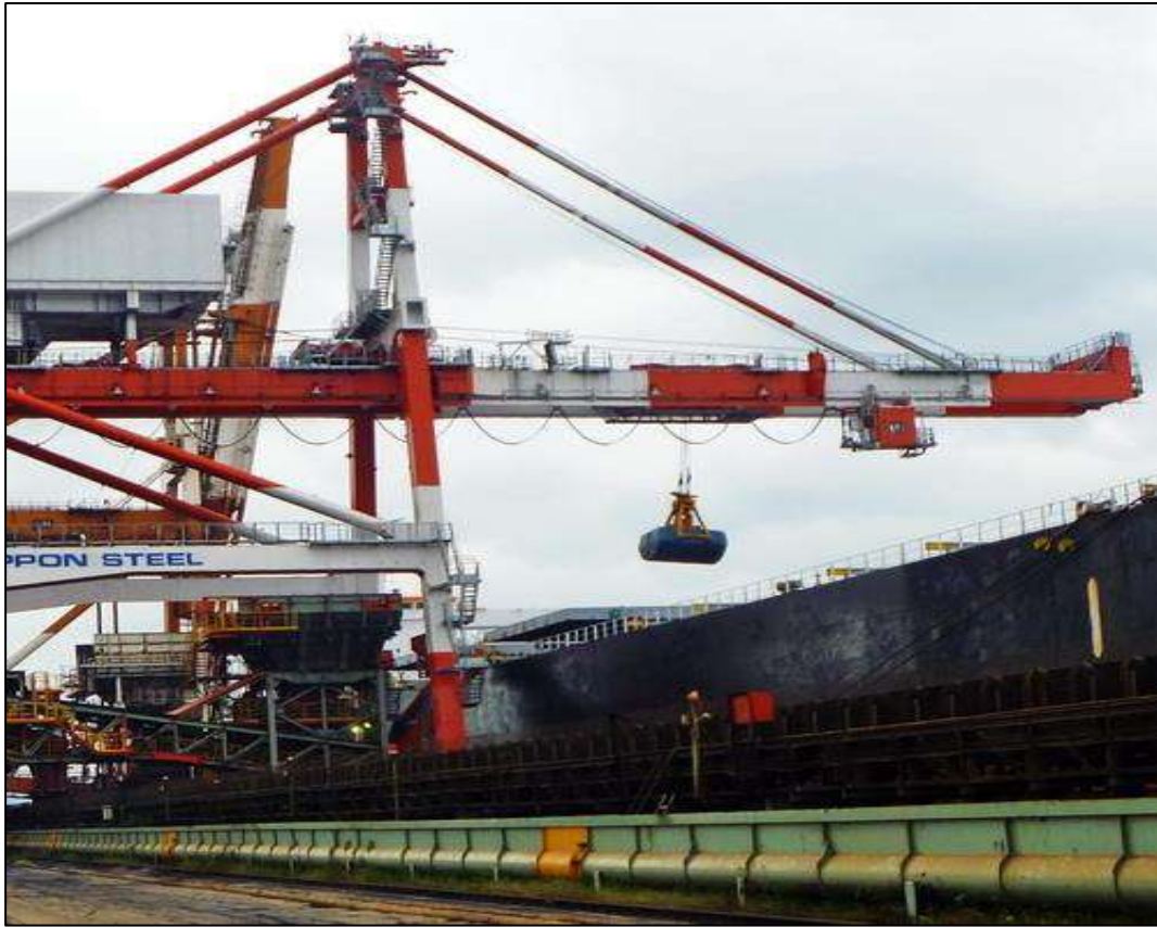
Figure 7.23 Typical Ship Unloader
