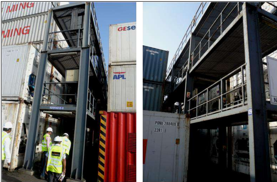
Figure 7.27 Typical Details of Reefer Stacks
