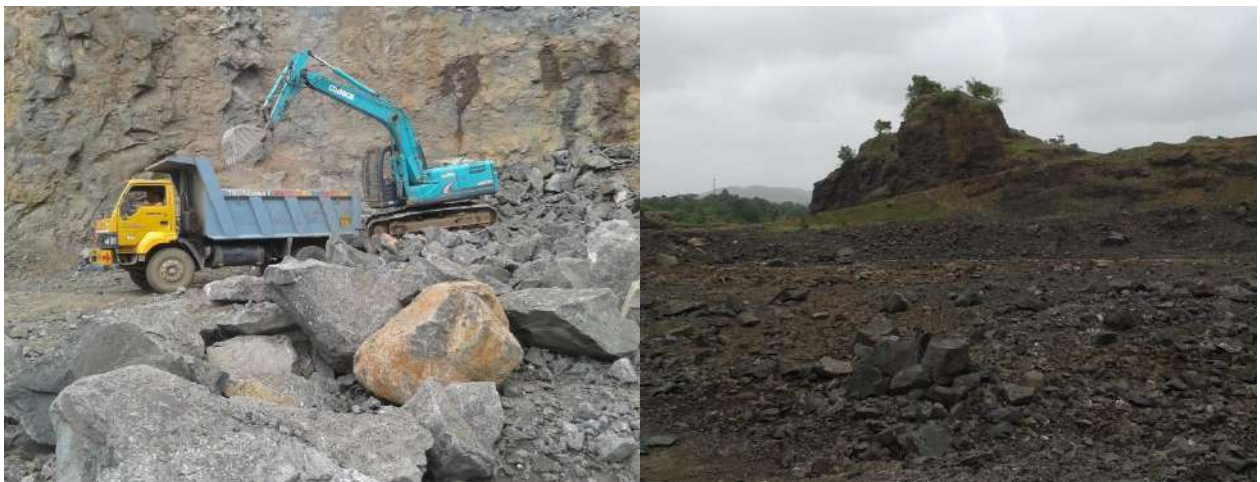
Figure 7.22 Existing Quarry site in Nagzari Village
