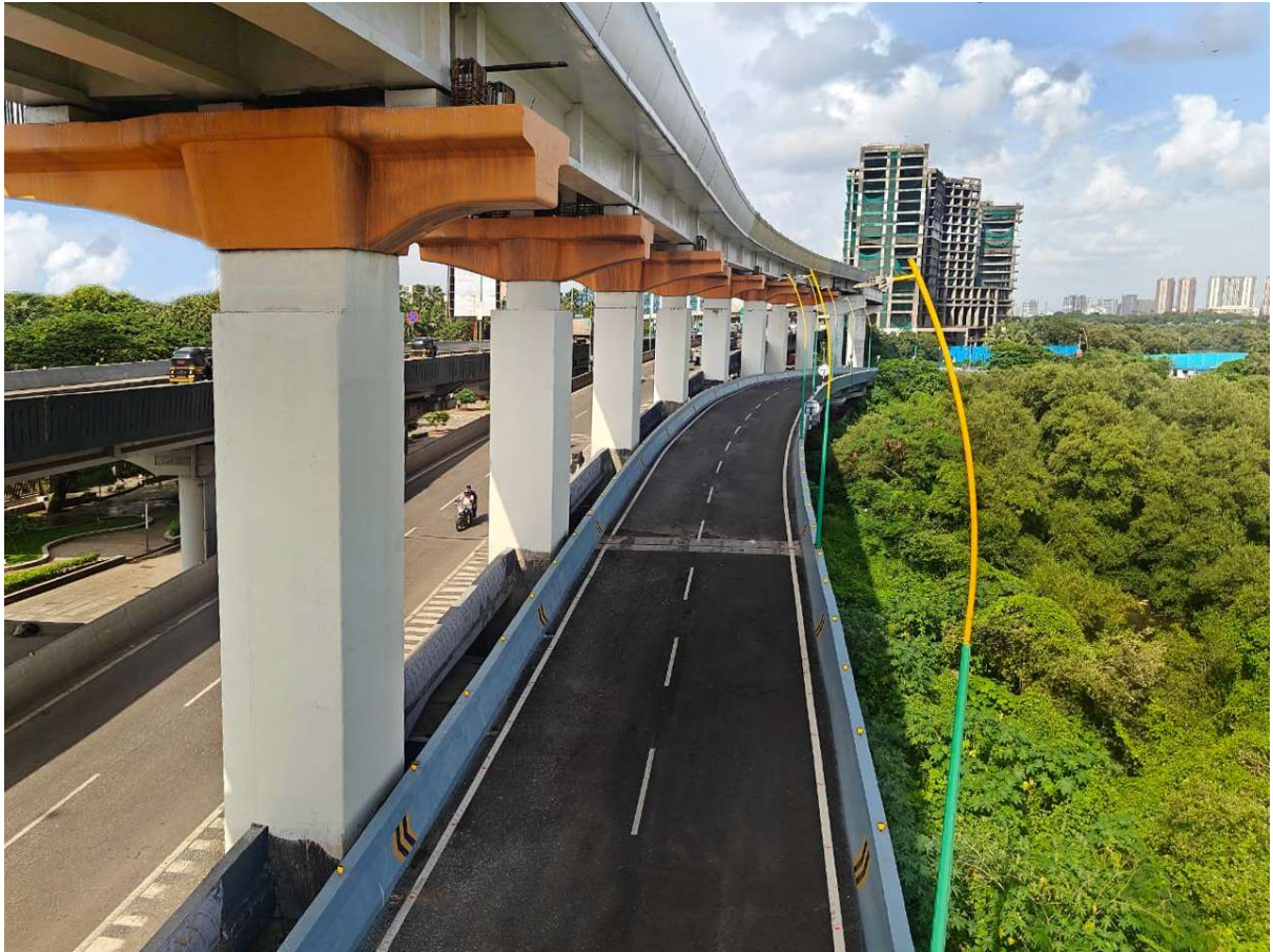
Kalanagar Flyover (Arm-D)
